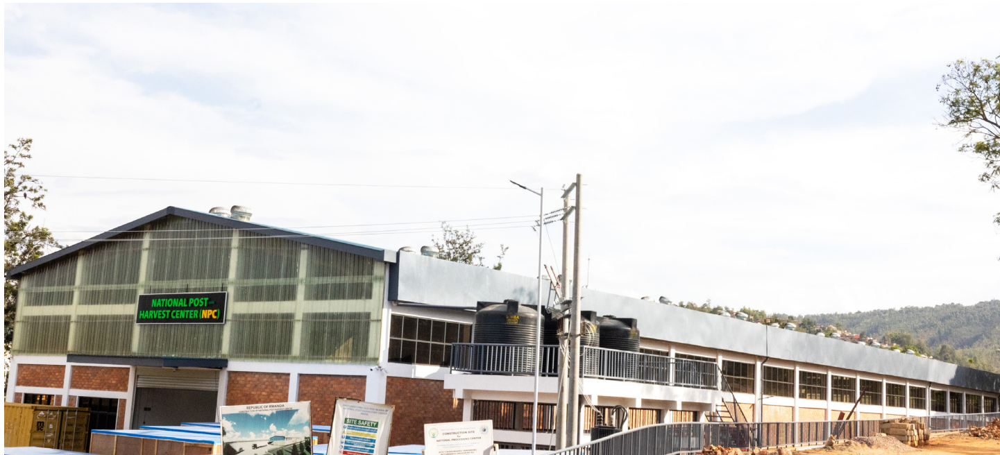
National Post-Harvest Center under construction
